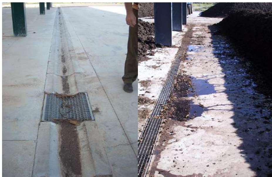
Figure 37. Examples of capture of leachates along the perimeter of the composting areas.
